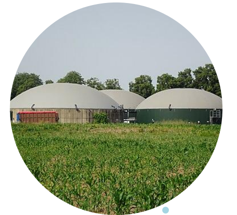
At anaerobic digestion facilities a biologic process in absence of oxygen takes place from which biogas (energy) is obtained
