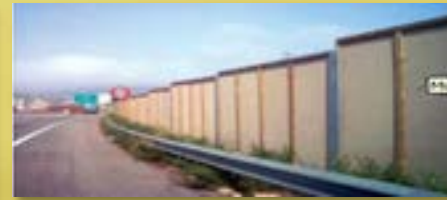
soundproof panels made with recycled carpet
